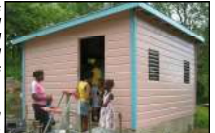
Charmaine & children see their new house nearing completion
